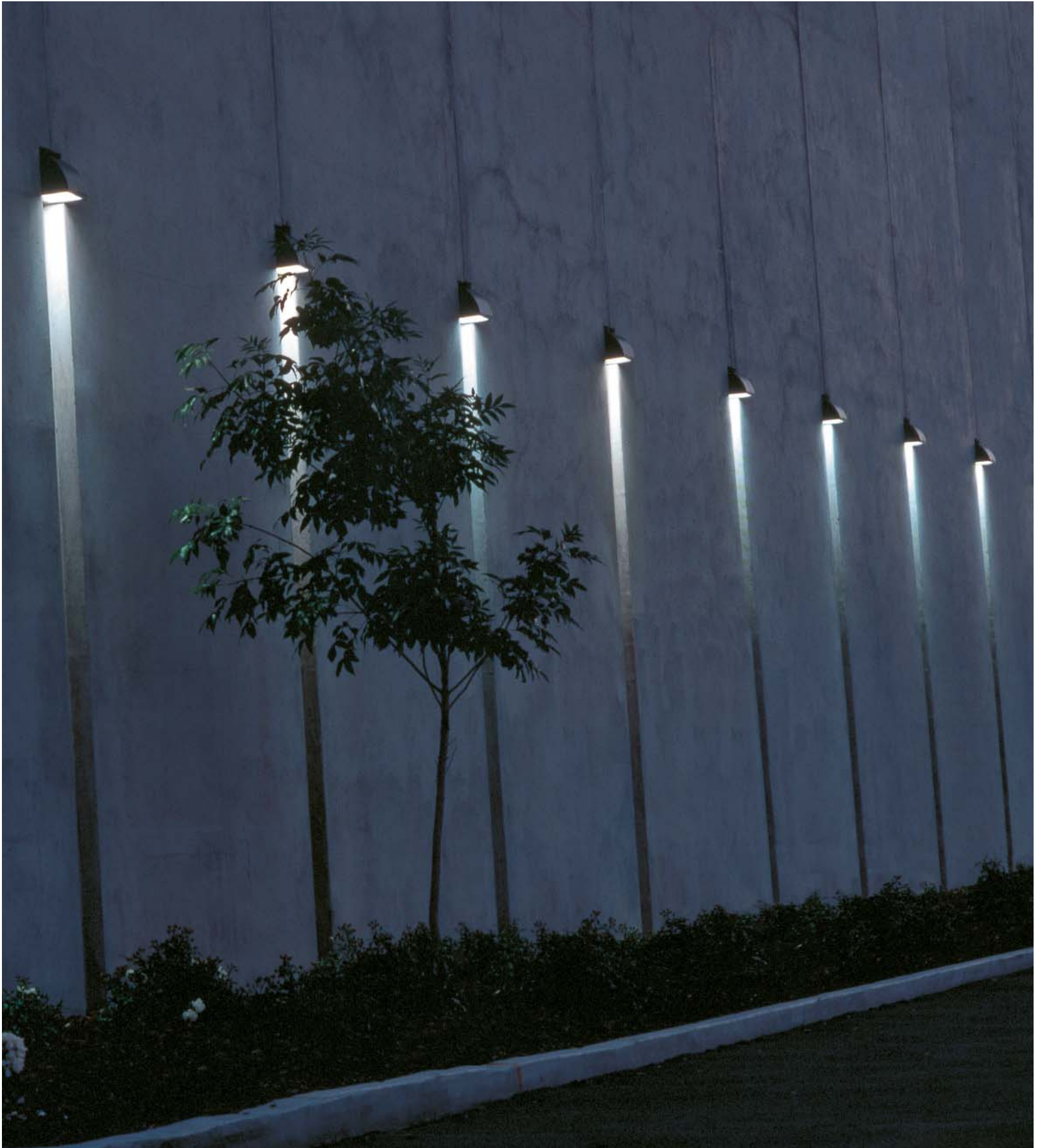
Christchurch Convention Centre. Christchurch (NZ). Architect: Warren & Mahoney. Lighting design: Beca Carter, Hollings & Ferner.
